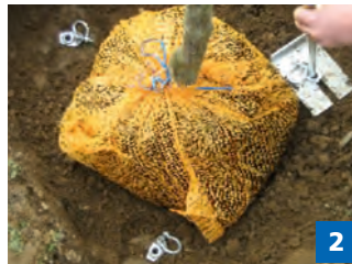
Installing the hammered anchors (see page 15).
