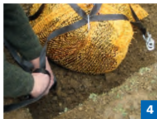
Installing the special hooks.
