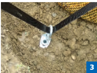
Installing the strap.
