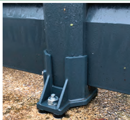
Bolt anchor for fence foot in concrete.
