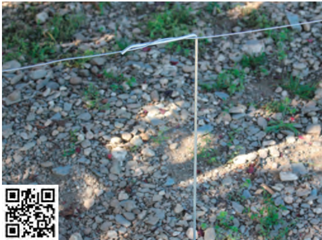
"1" shape stake into the ground and on the wire. Scan to view the video.
