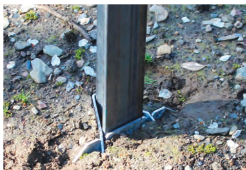
"T" post with reinforcement cross.
