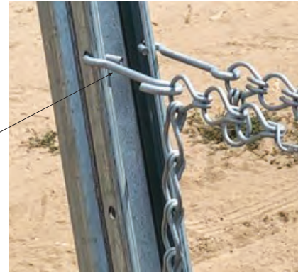
Ties hook on post with side holes.
