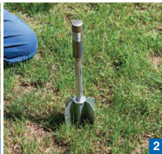
Driving in the hammered anchor.
