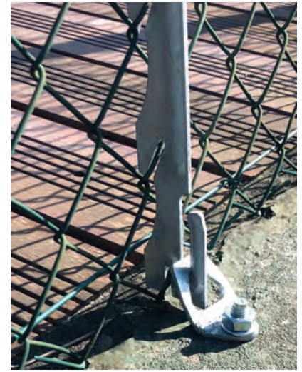
Multiple wire holder in concrete.
