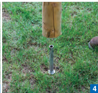
Fitting of the wooden post on the hammered anchor.
