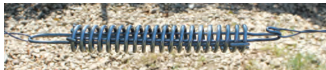
Compensating spring installed on the moveable wire.
