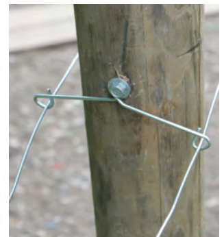
Spring wire spreader on wooden post.
