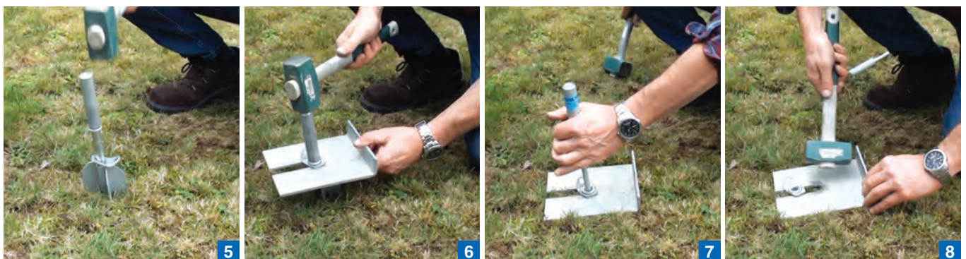
5 Start to drive the anchor in the ground with the driving tool.
