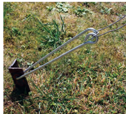
Twin extension on angled post.
