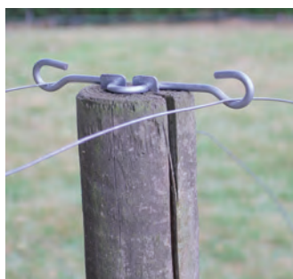
Moveable wires guide on wooden post.
