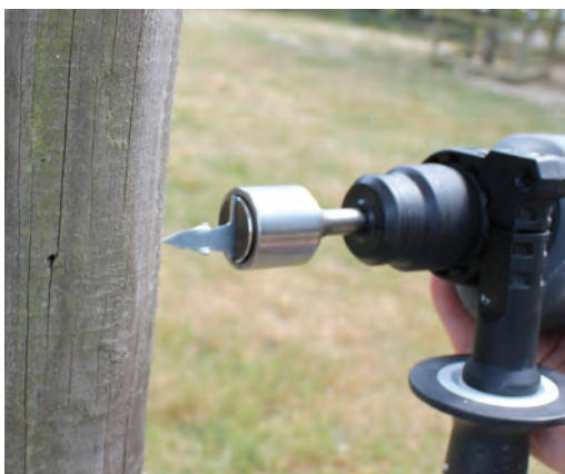
Installation of spreader tips with nailer tool.
