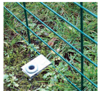
Single wire holder with hammered anchor in the ground.
