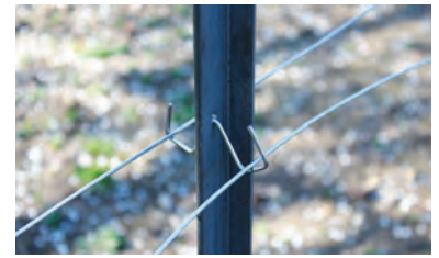
Symmetrical spreader in position on T post.
