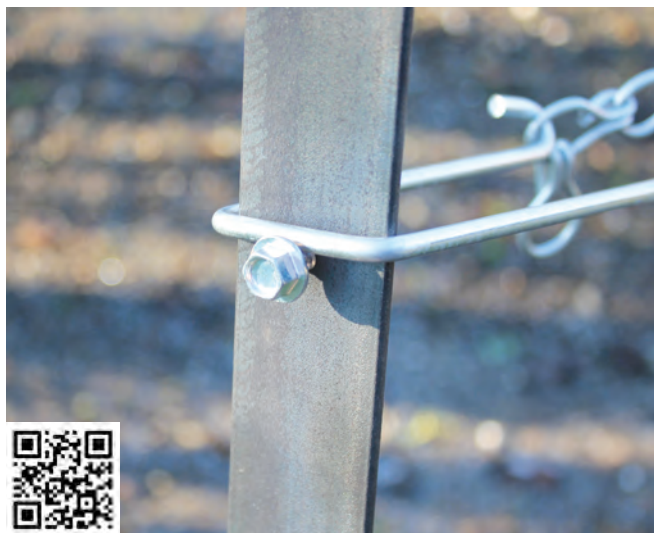
Square tie with supporting screw on metal post.
