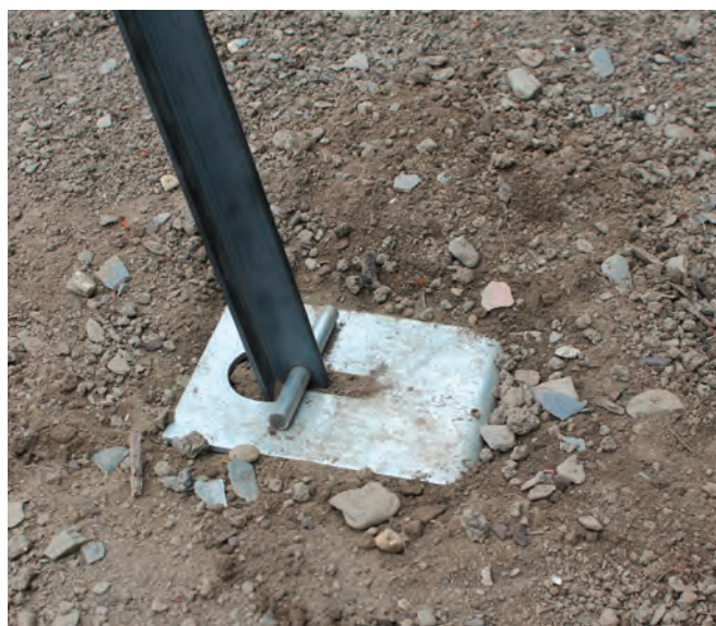
Anti-sinking plate with "T" post.
