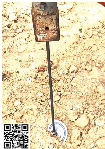
Fixgrip anchor during driving. Scan to view the video.
