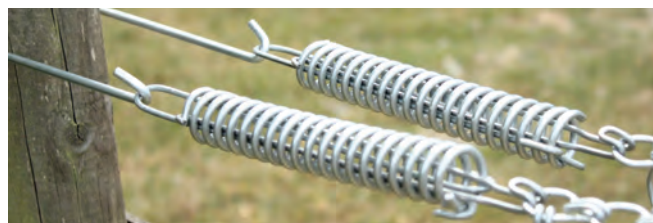
Compensating spring installed on the end ties.
