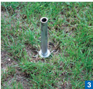
Deploy rods using the sleeve and the split plate.
